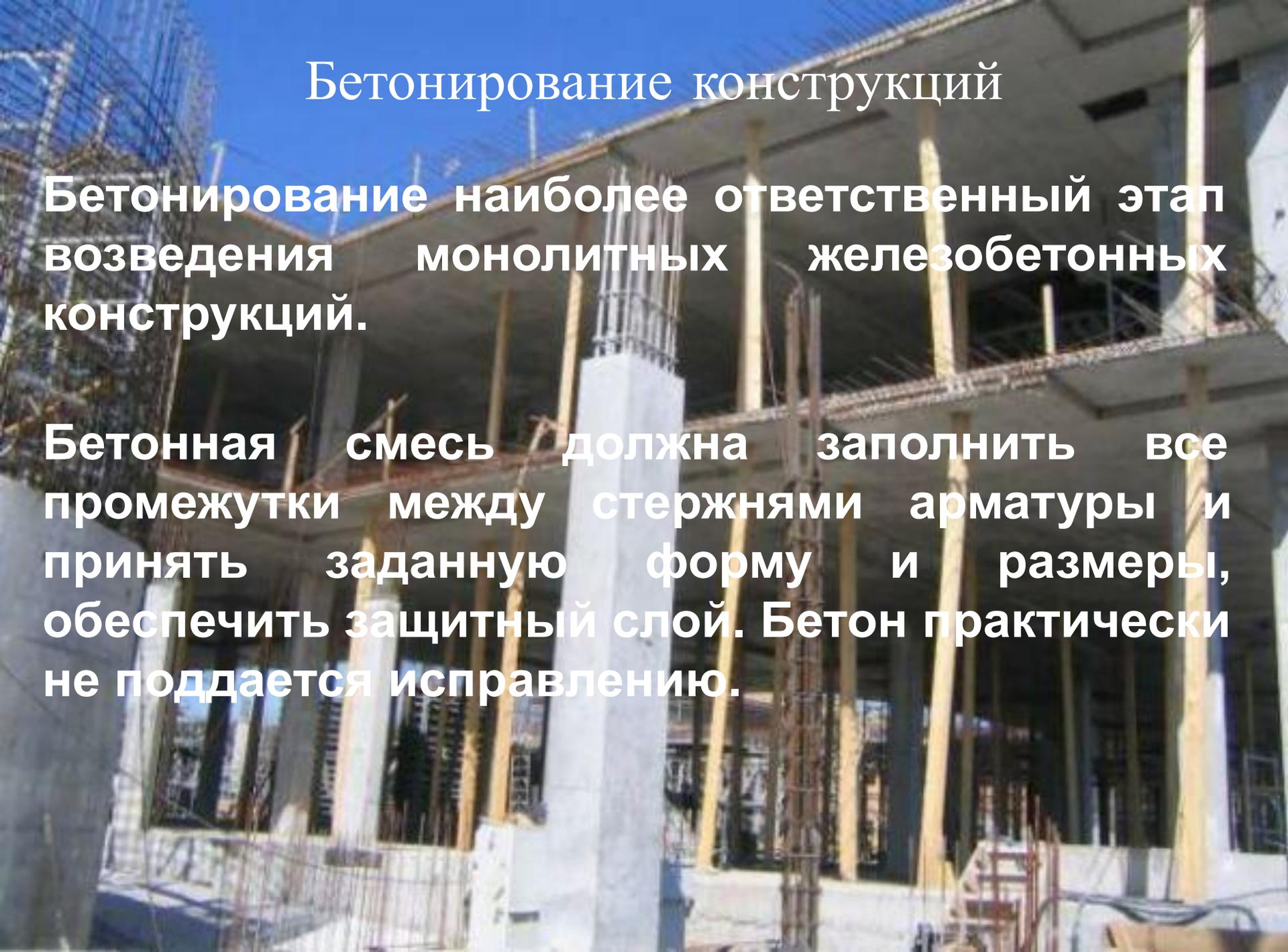
A photograph of a construction site during the concrete pouring phase. A vertical concrete column is being formed, with a dense network of rebar visible at the top. The structure is surrounded by wooden formwork and scaffolding. The sky is clear and blue.
