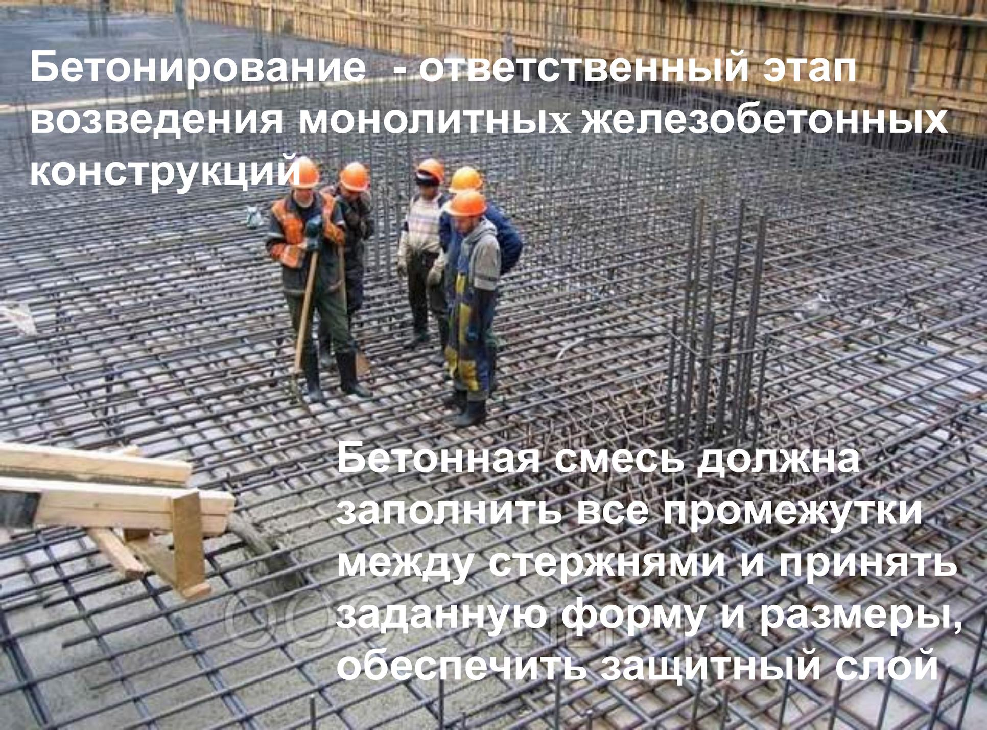
A photograph showing several construction workers in orange hard hats and safety vests standing on a dense grid of steel reinforcement bars (rebar) laid out on a construction site. The workers are positioned in the middle ground, looking towards the camera. The background shows a wooden formwork structure. The overall scene is a typical construction site for a concrete slab.
