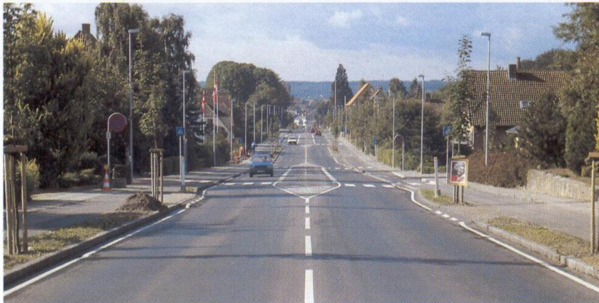
*The traffic island shields off the left-turn lane and provides for safer crossing of the road.*
