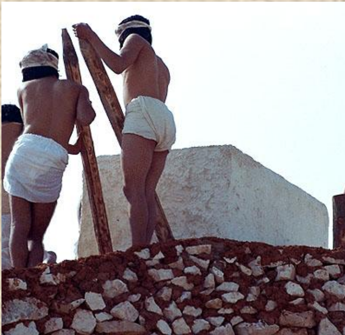
Rocking a block into position
