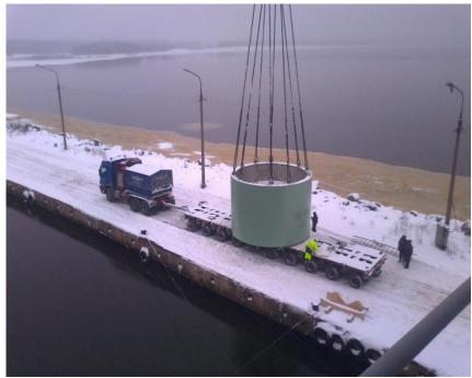
The heaviest items (weight up to 161 MT) were delivered by floating crane and then this crane reloaded equipment on trucks.
