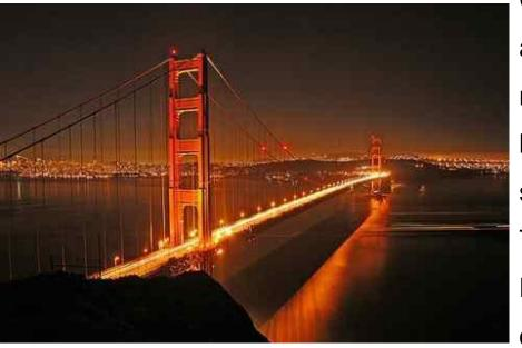
Constructions on the bridge began in 1933 and were completed in 1937. The bridge rises 230 m above the water. With its total length of 1970 meters it was the longest suspension bridge in the world until 1964. The bridge is part of the United States Highway 101, has six lanes and a footpath on each side.
