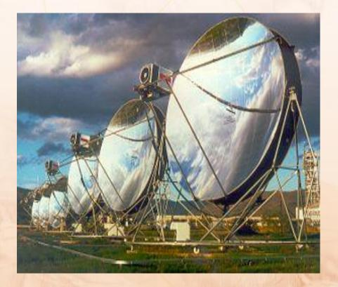
A parabolic dish and Stirling engine system, which concentrates solar energy to produce useful solar power.
