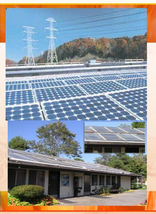
Active solar techniques include the use of photovoltaic panels, solar thermal collectors, with electrical or mechanical equipment, to convert sunlight into useful outputs.
