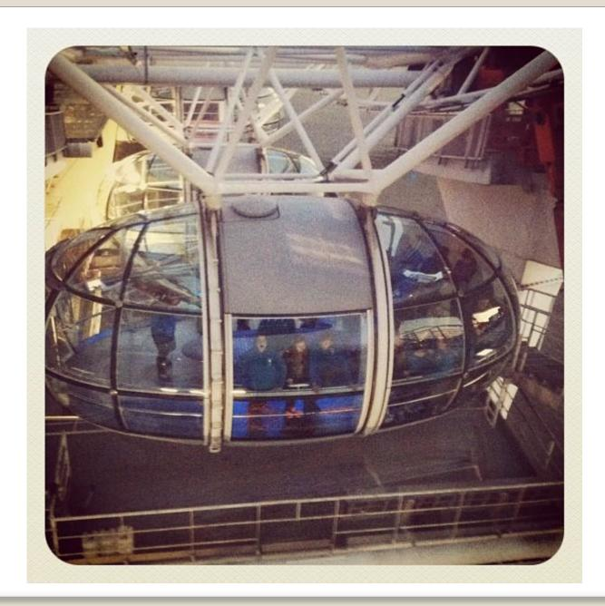
The wheel rotates at 26 cm (10 in) per second (about 0.9 km/h or 0.6 mph) so that one revolution takes about 30 minutes. It does not usually stop to take on passengers; the rotation rate is slow enough to allow passengers to walk on and off the moving capsules at ground level. It is, however, stopped to allow disabled or elderly passengers time to embark and disembark safely.
