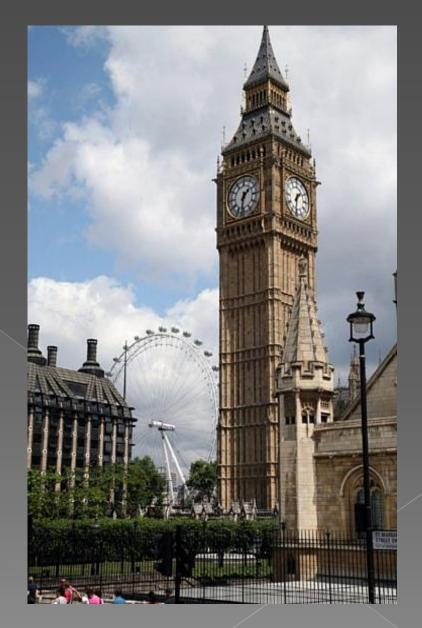
The clock and dials were designed by Augustus Pugin. The clock dials are set in an iron frame 23 feet (7 m) in diameter, supporting 312 pieces of opal glass, rather like a stained-glass window. Some of the glass pieces may be removed for inspection of the hands. The surround of the dials is gilded. At the base of each clock dial in gilt letters is the Latin inscription: "DOMINE SALVAM FAC **REGINAM NOSTRAM** VICTORIAM PRIMAM". (O Lord, keep safe our Queen Victoria the First).
